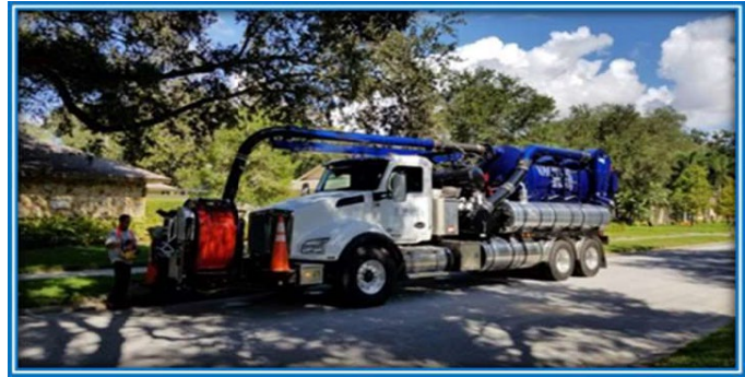
Stormwater Outfall Construction
