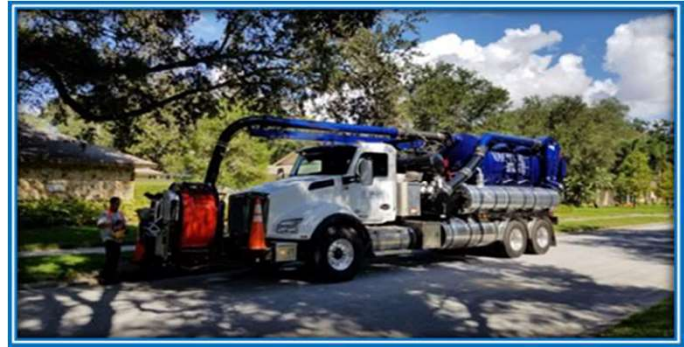
Stormwater Outfall Construction
