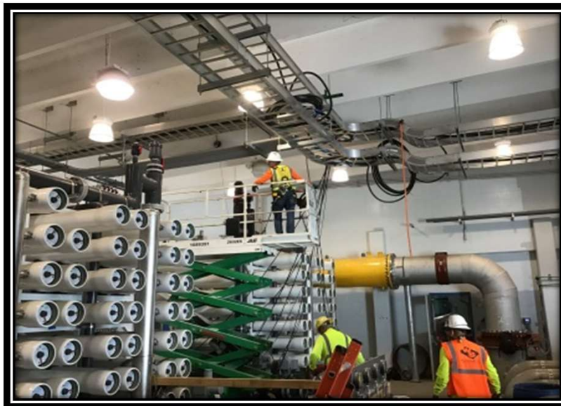
Reverse Osmosis Water Treatment Plant - Reconstruction / Restoration Project
