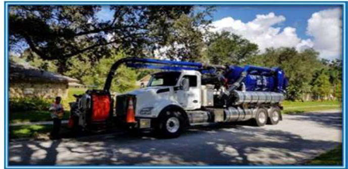
Stormwater Outfall Construction
