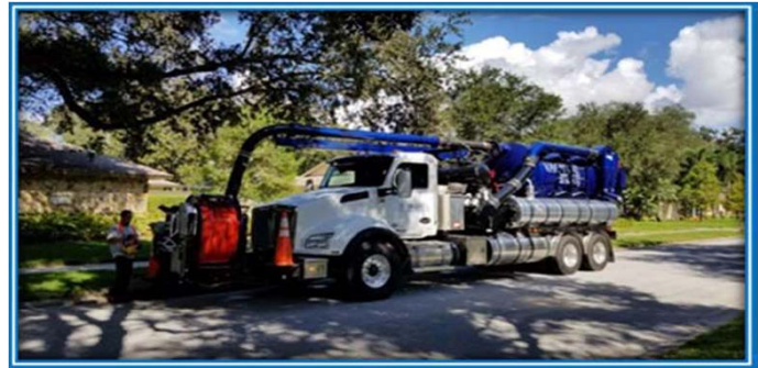
Stormwater Outfall Construction
