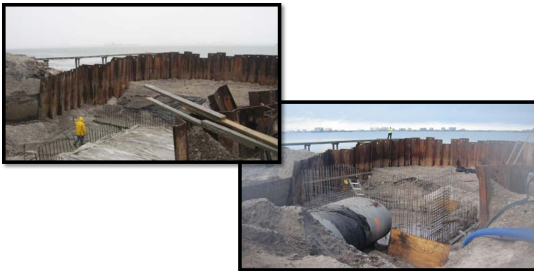
Stormwater Outfall Construction
