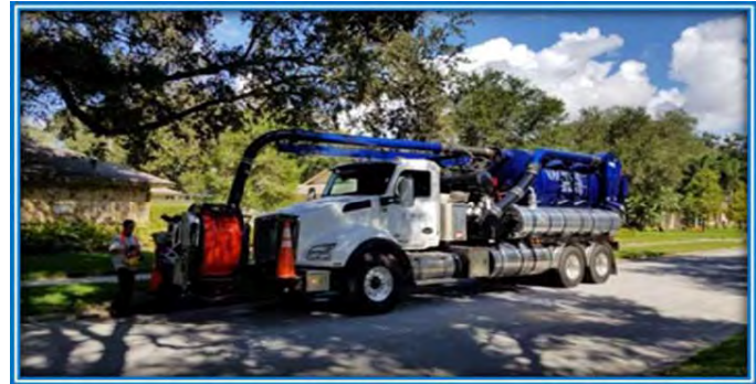
Stormwater Outfall Construction
