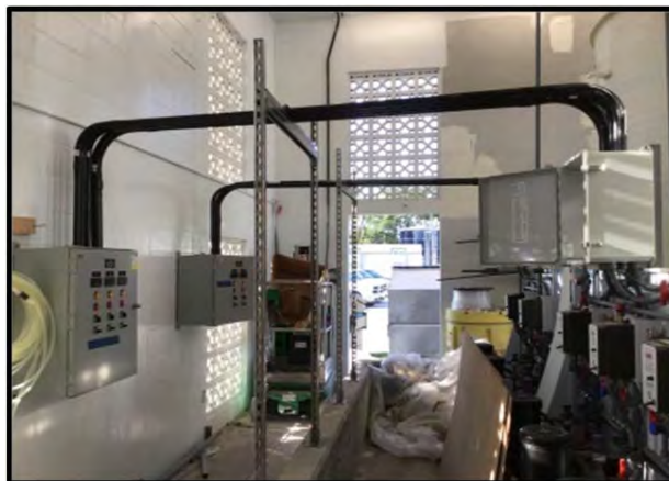
Reverse Osmosis Water Treatment Plant - Reconstruction / Restoration Project
