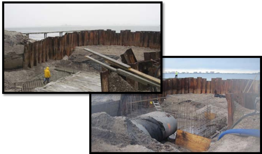
Stormwater Outfall Construction
