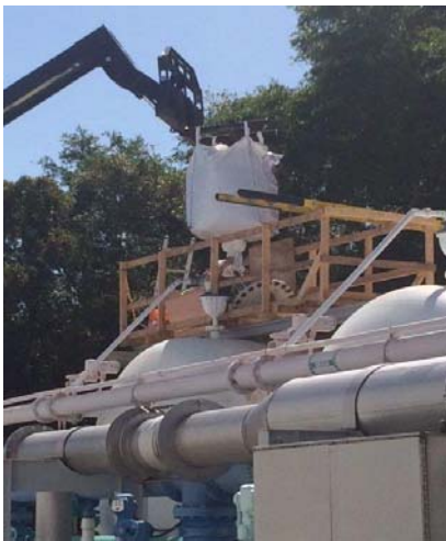
Greensand filter media replacement project
