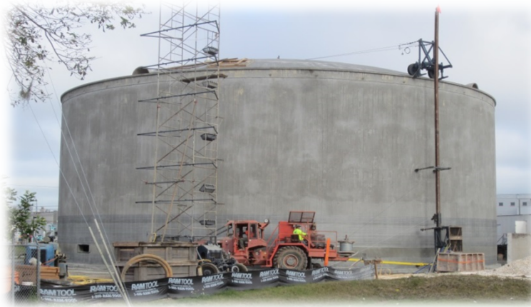
Wastewater Treatment Plant - Reclaimed Water Ground Storage Tank under construction
