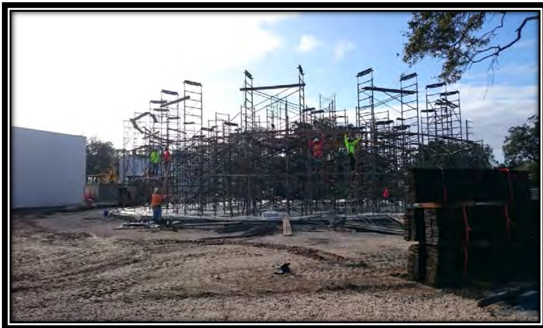
Wastewater Treatment Plant - Reclaimed Water Ground Storage Tank under construction
