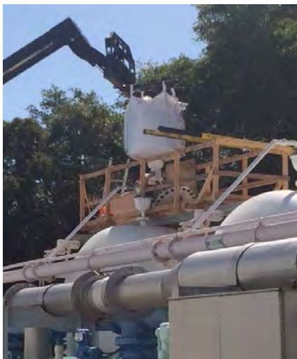
Greensand filter media replacement project
