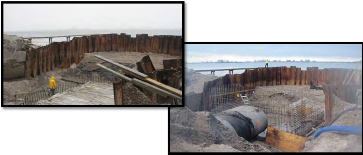
Stormwater Outfall Construction
