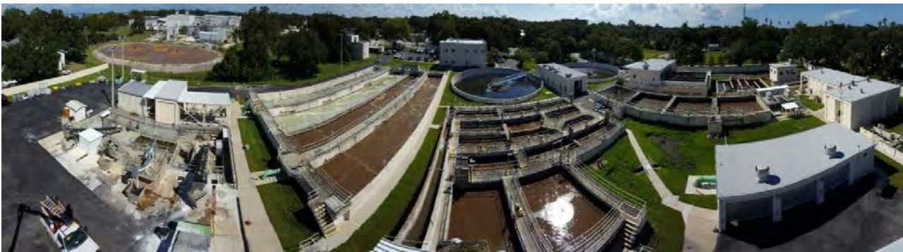
Wastewater Treatment Plant
