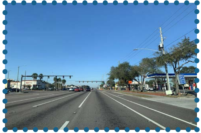
Bike Lane on SR 580
