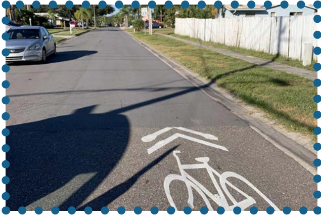
Shared Lane Marking on McCarty Street
