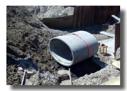
[Image 7-3] Drainage Pipe for Stormwater
